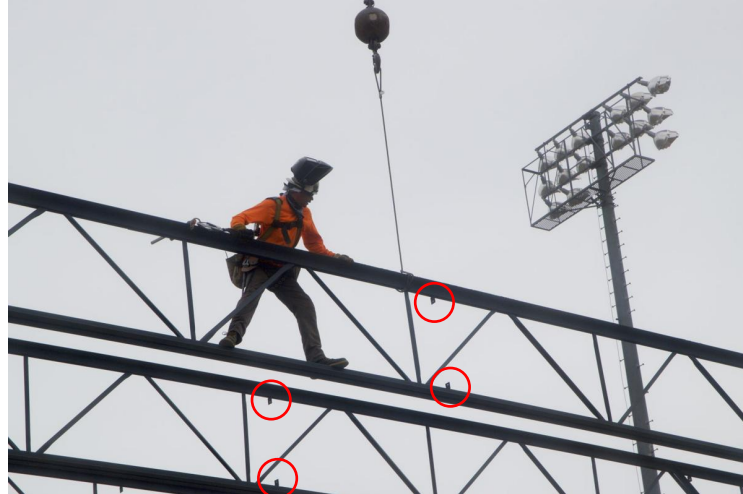
Figure 26. Erection of joist (Cole, 2018)
