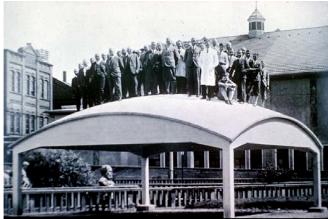
Figure 5. Dischinger shell loaded by the Dyckerhoff and Widmann engineers in 1932 in Weisbaden-Biebrich, Germany (Hines & Billington, 2004)
