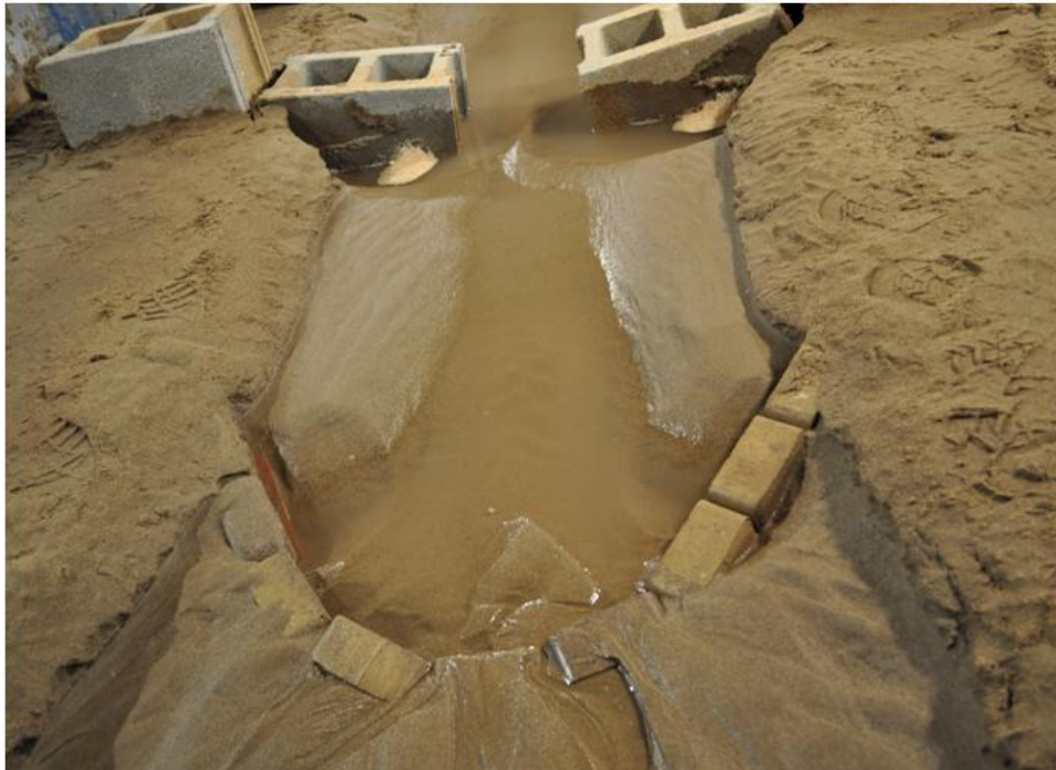
Figure 30 – Photograph of the upstream cross vane after trial 4 (facing downstream).
