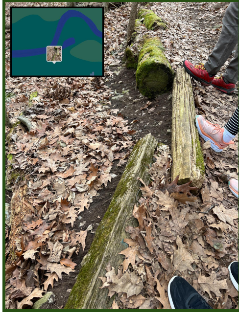
Figure 7: Example of switchback infrastructure on Dale's Ridge Trail. Noticeable moss and movement of logs due to erosion are visible throughout the entire section (map taken from iPhone)
