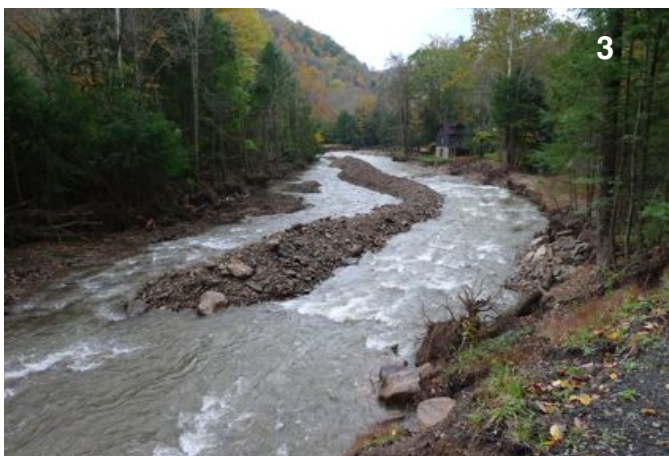
3. Removal of gravel point bar, realignment of main flow channel, regrading of channel slope and width. (late September 2011).
