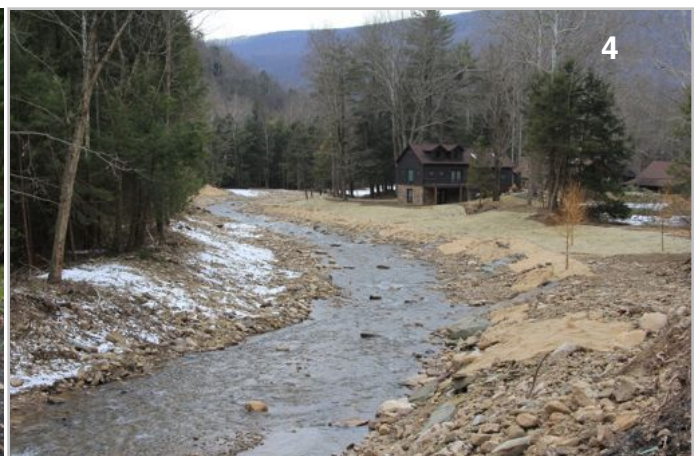
4. Reworking of channel banks, installation of rock veins on meander bend, regrading and armoring of channel banks. (October, 2011)
